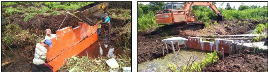
Fig. 5. Implementation Process of Composite Canal Blocking Module
