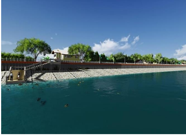
Fig. 8. Front view of the mitigation system.
