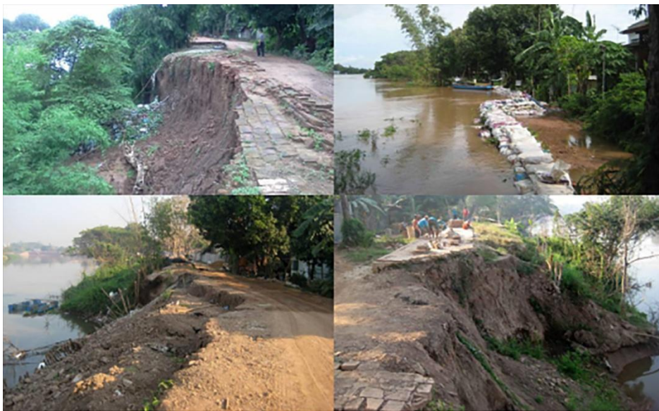
Fig. 3. Consequences from the river erosion and flooding event in 2011.
