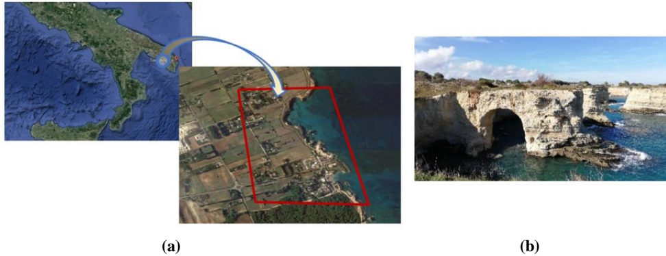
Fig. 2. Identification of the study area called “A” (approximate geographic coordinates: 40^{\circ}15'16.30''\text{N} , 18^{\circ}26'38.68''\text{E} , WGS84) (a) and panorama image of the cliff (b).
