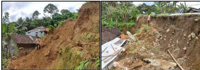
Fig. 6. Slope 1 (LR 1), left, and Slope 2 (LR 2), right.
