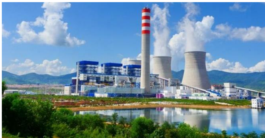
Fig 1. Hongsa coal-fired power plant in Sayabouri province, Lao People's Democratic Republic (Source of data:
