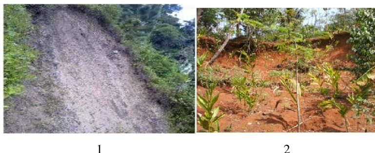
Fig.9. Landslide appearance photos in 1.Krajan Village, 2. Village Semedo, (Source: Suwarno, 2014)
