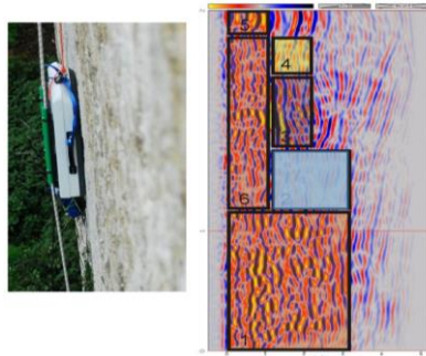
Fig. 14 Section done with the GPR
