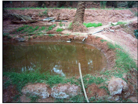
Fig. 4 Basin water storage called Madjen
