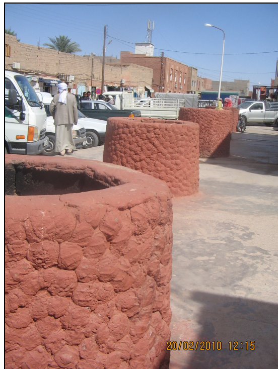
Fig. 2 Ventilation shaft of foggara through the Adrar city
