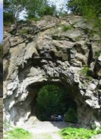
Fig. 9 Rail tunnel built – Tișiței Gorges
