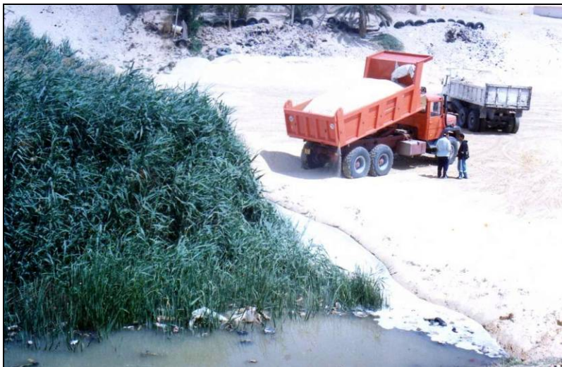
Fig. 11 Backfilling operation Ghouts (photography Remini B., 2002)
